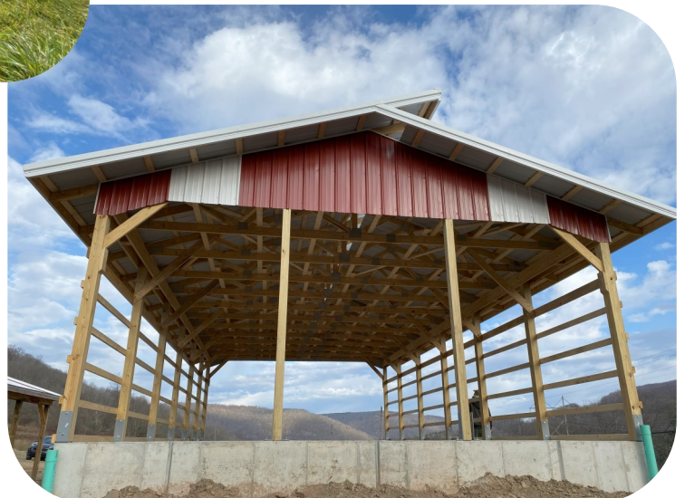
Roofed manure stacking facility
