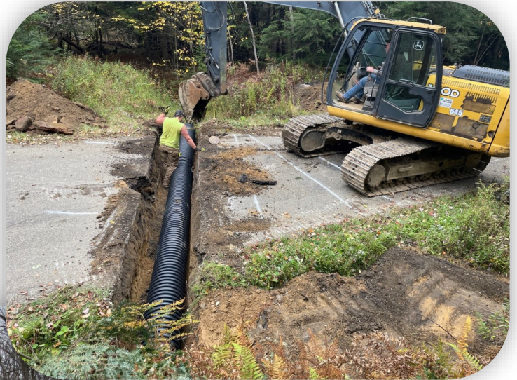
Above: Taintor Road, Lafayette Township, during project construction. Picture shows installation of a new crosspipe.
