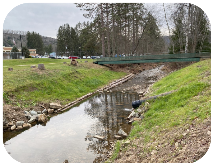
After : Streambank stabilized with a modified mudstill
